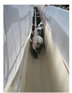
In a series of tests made by the Bureau of Reclamation for the EPA, Zebron coatings showed no defects when immersed in oxygenated wastewater for periods of 28 months. Of 13 products tested, it was one of only two products to show no defect throughout testing.
