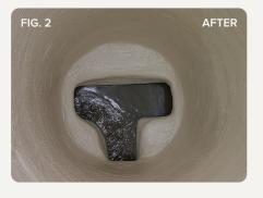
The low permeability of ZEBRON® makes it ideal for protecting sewage systems from hydrogen sulfide gas and for protecting metal surfaces from corrosive atmospheres.
