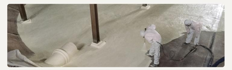
ZEBRON® #386/9000 and #486/9000 meet the ANSI/NSF Standard 61, Section 5, Barrier Materials testing requirements for use in potable water. Certification documentation is available upon request.
